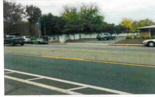
3 LOOKING EAST AT SITE FROM POLE LINE ROAD
